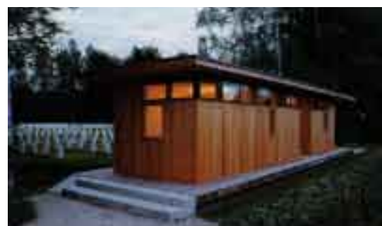
frediani gasser_service building
