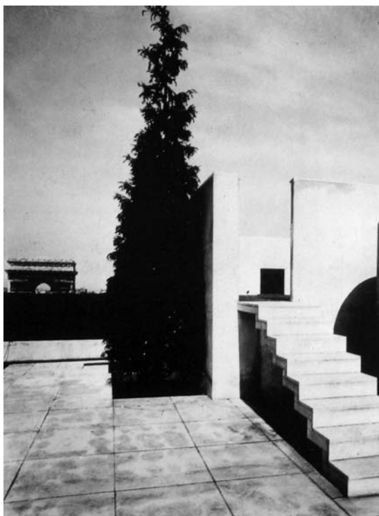
Figure 6 Le Corbusier, Bestegui Apartment, Paris 1929-31 (from Rassegna: Cemento, 1992(49), p. 34
