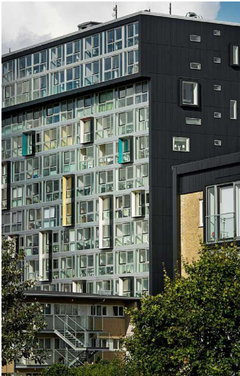
_Glass and steel for the renewed north and south facades
